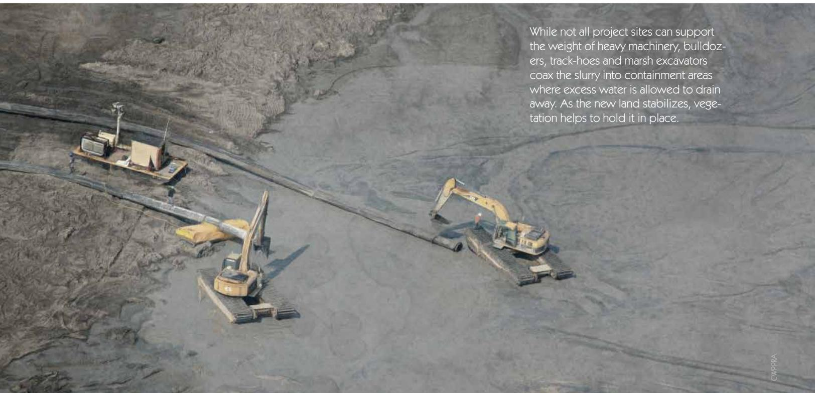
While not all project sites can support the weight of heavy machinery, bulldozers, track-hoes and marsh excavators coax the slurry into containment areas where excess water is allowed to drain away. As the new land stabilizes, vegetation helps to hold it in place.
